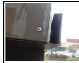
Missing Retainer
