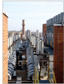
PHOTO A. The roof of Jordan Hall was covered with 200 small exhaust fans, which presented a maintenance challenge in the form of continuous roof leaks where exhaust risers connected to the fans. The high-dilution-exhaust-fan system that replaced the fans can be seen on the far right.
