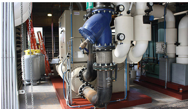
FIGURE 3. This new 700-ton (oil free) chiller utilizes magnetic bearing technology which eliminates bearing surface wear for high-efficiency operation and extended life of the machine.
