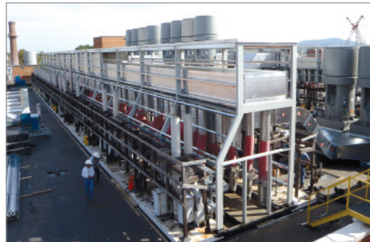
PHOTO B. Central exhaust system under construction with new manifold and existing fans.
