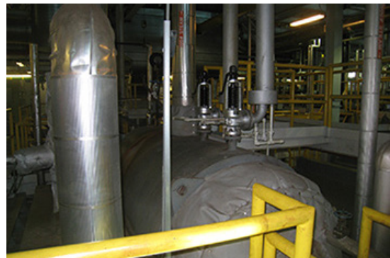
High-pressure steam boiler with multiple relief valves and drip-pan elbow.
