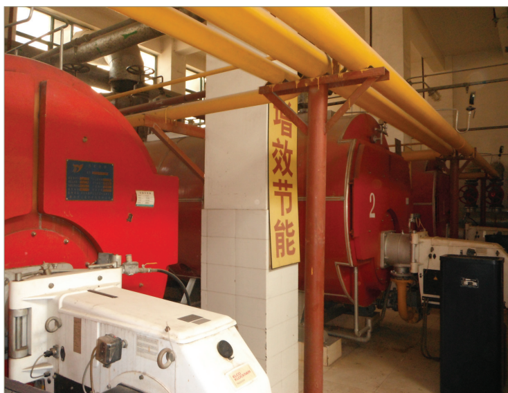
Firtube boilers in the Xi’an district energy system
