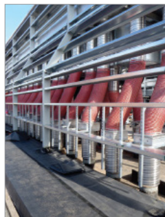
PHOTO C. New exhaust-duct manifold.
