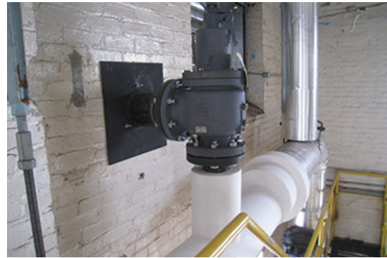
Steam application with no drip-pan elbow and outlet is restricted from thermal growth.
