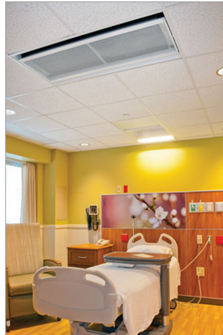
A patient room with chilled-beam technology.
