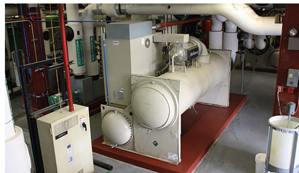
FIGURE 4. Magnetic bearing technology when applied to the design of the conventional centrifugal compressor gives way to a smaller, quieter compressor as seen here in the magnetic bearing compressor installed at Mount Vernon Hospital
