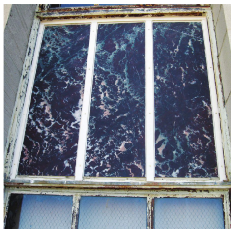
This is the original marble in the framed opening. Not only is there a crack in the panel to the right along one of the natural soft veins in the stone, but the marble had also lost its luster and burgundy color.
