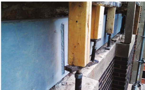
A before and after photo of the repair performed at a steel spandrel beam. The moment splice plate behind the screw jacks is needed for the new steel member installation.
