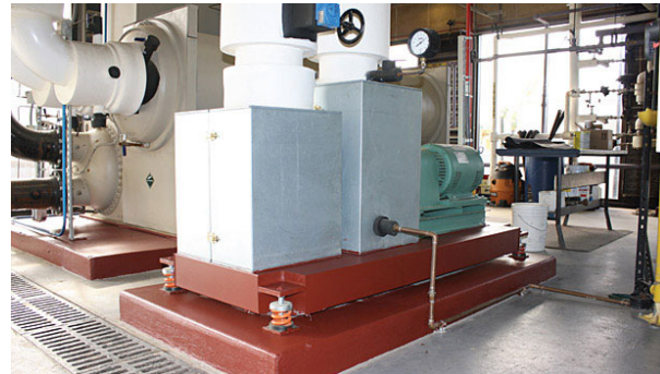
FIGURE 2. New variable speed primary pumps were installed for a variable primary/variable secondary chilled water distribution for reduced pumping energy.
