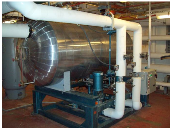
Figure 6 – A new condensate tank and pump set normally work in parallel with the original condensate system yet the older receiver to be taken off line for inspection and maintenance while the plant remains in operation.
