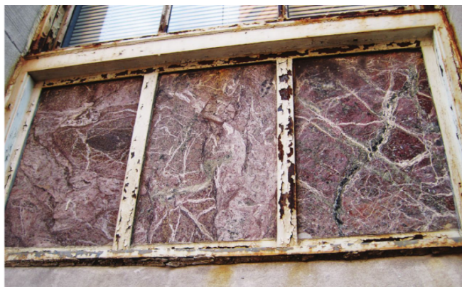
This is the original marble in the framed opening. Not only is there a crack in the panel to the right along one of the natural soft veins in the stone, but the marble had also lost its luster and burgundy color.
