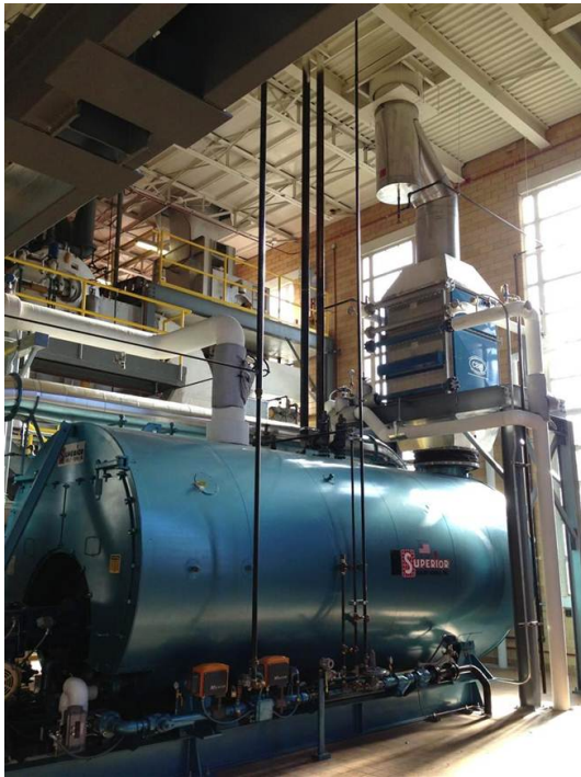
Figure 8 – Boiler three occupies a slot in the plant originally designed for a unit more than three times its size. The new boiler is a perfect fit to add capacity and improve plant efficiency.
