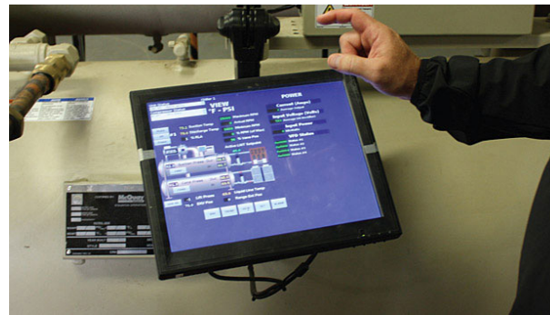
FIGURE 6. On board microprocessor controller and unit-mounted touchscreen panel with full system graphics provides the plant operators with a view of the chiller parameters and design set points at a glance.
