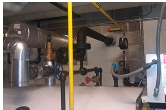
Low-pressure steam boiler with drip-pan elbow. Vent pipe is not supported.
